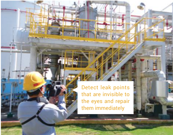
Use Gas Find IR for on-site detection
