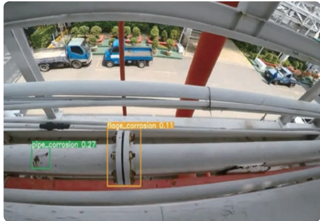
Image recognition of defects in process pipe flanges and pipelines
