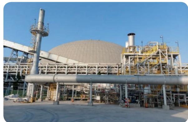
Replacement of old control equipment with new ones
