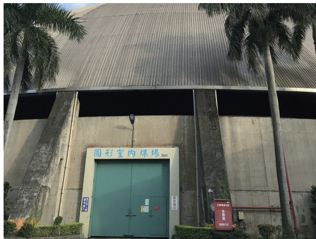
The Closed Coal Bunker
