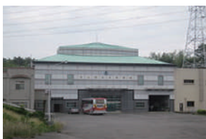
Wushantou Power Plant
