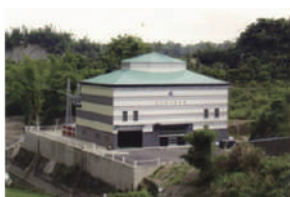
Xikou Power Plant
