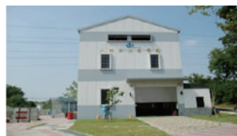
Hatta Power Plant
