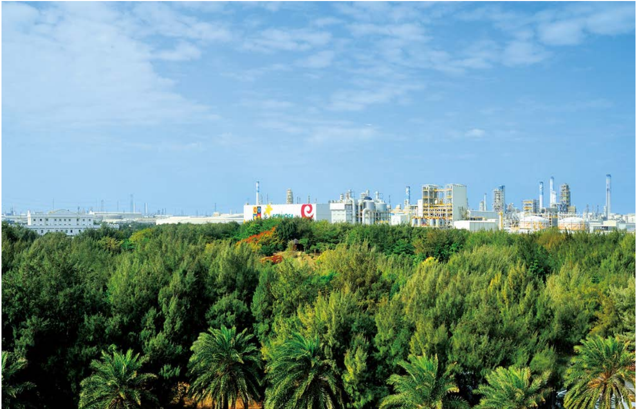
..... FPG Mailiao Eco-Industrial Complex
