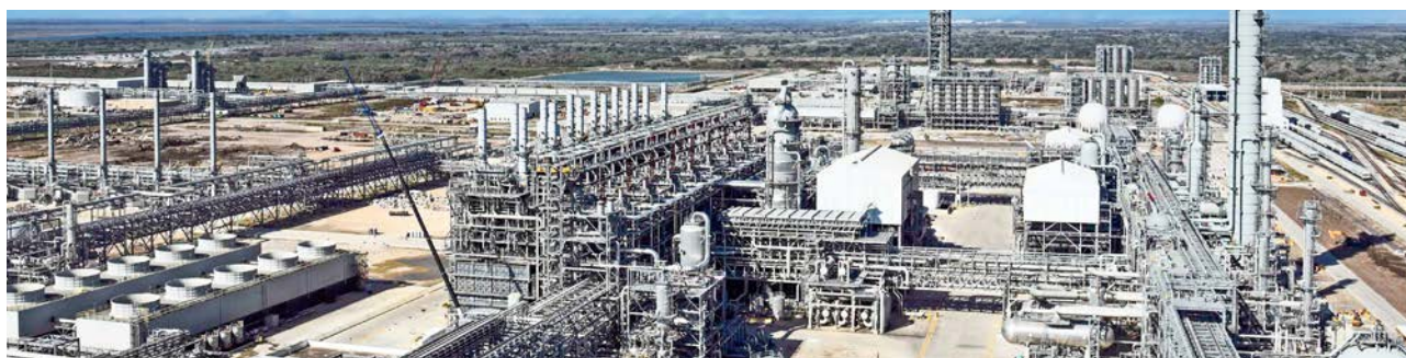
..... Olefins III Plant in Point Comfort, TX
