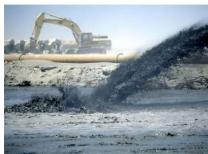
Pumping sand to fill the sea
