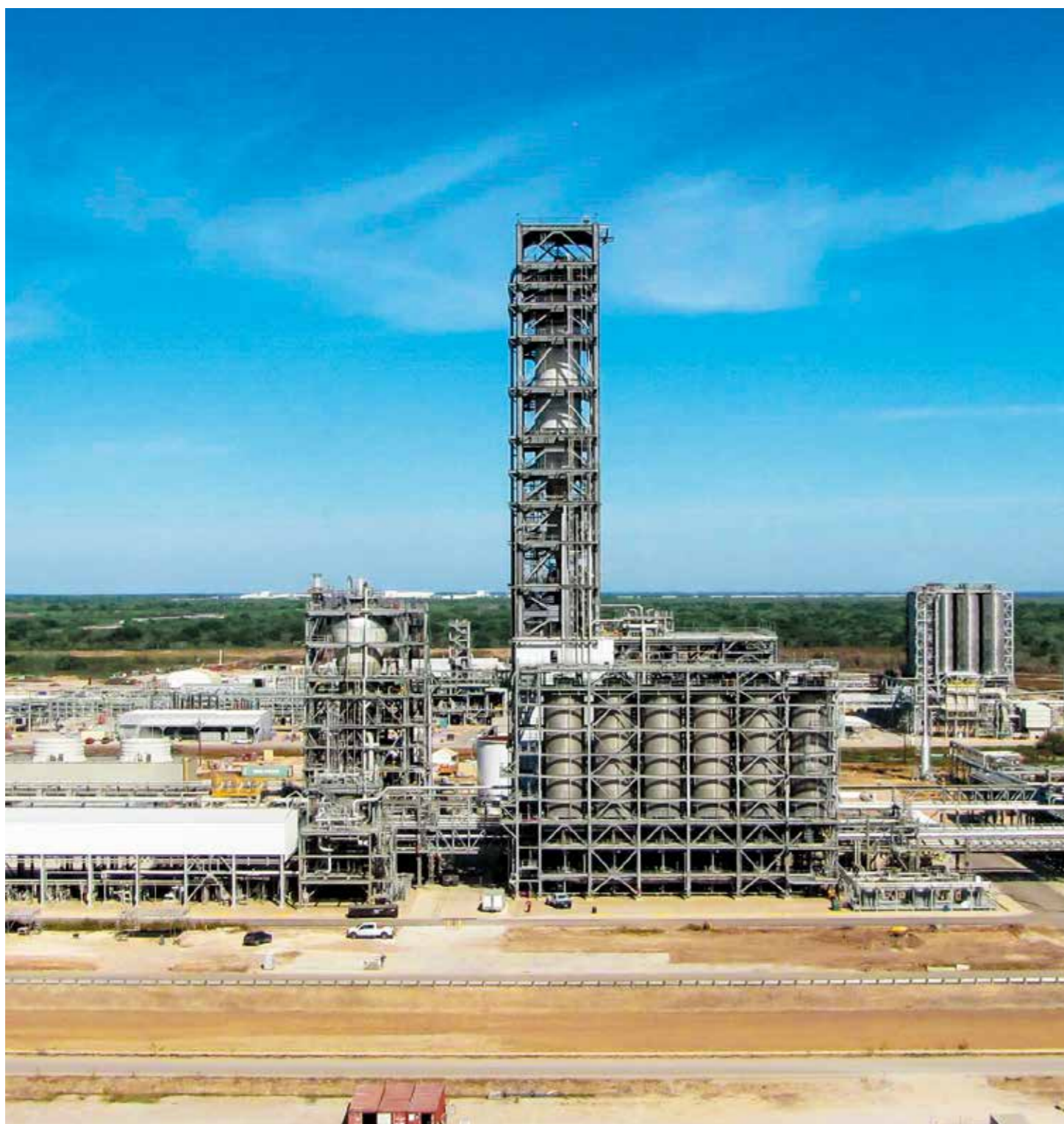
| New LDPE Plant in Construction |
