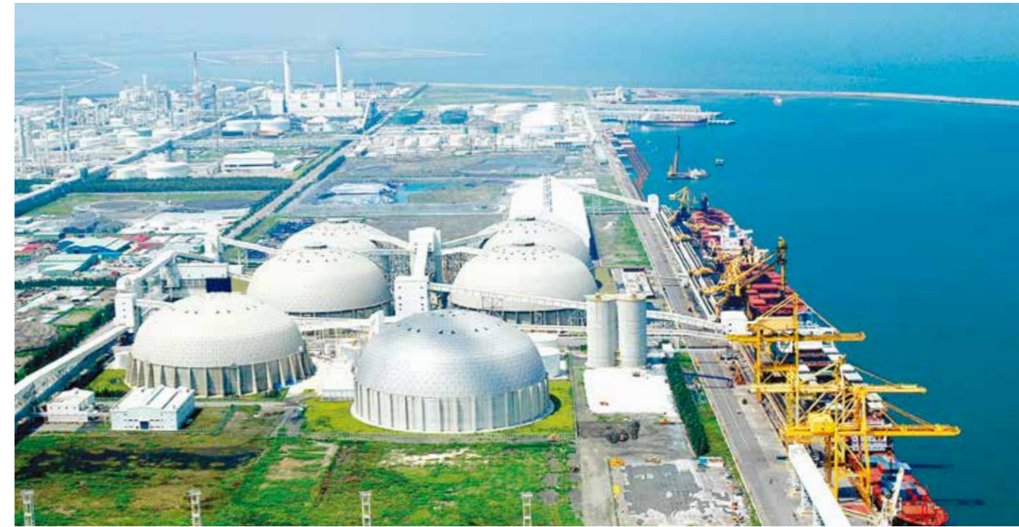
Completion of Shore Power System
