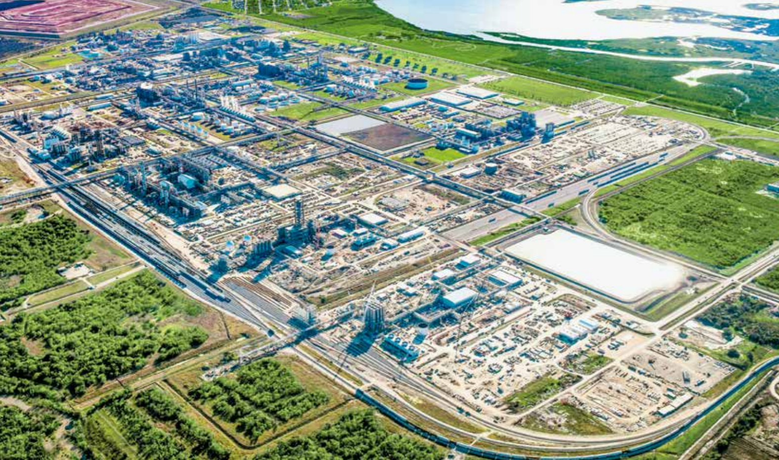
Aerial Bird View of Point Comfort Complex, TX
