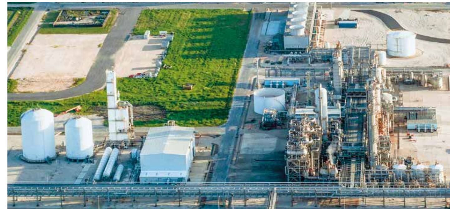
EG Plant, Texas
