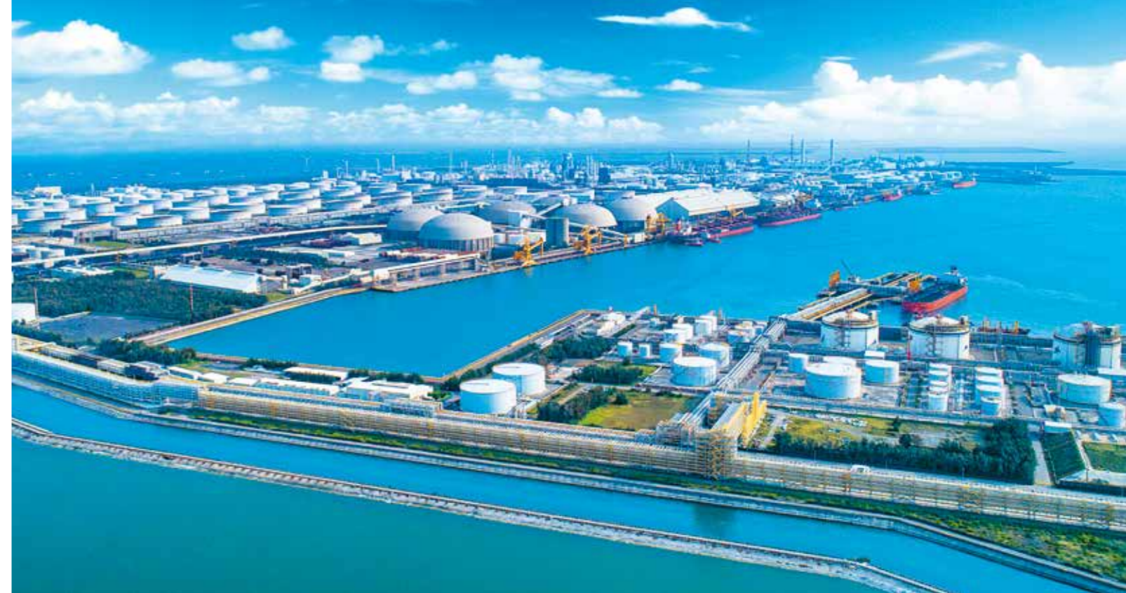
Mailiao Harbor Building highly automated pipeline transmission system & high-pressure shore power system
