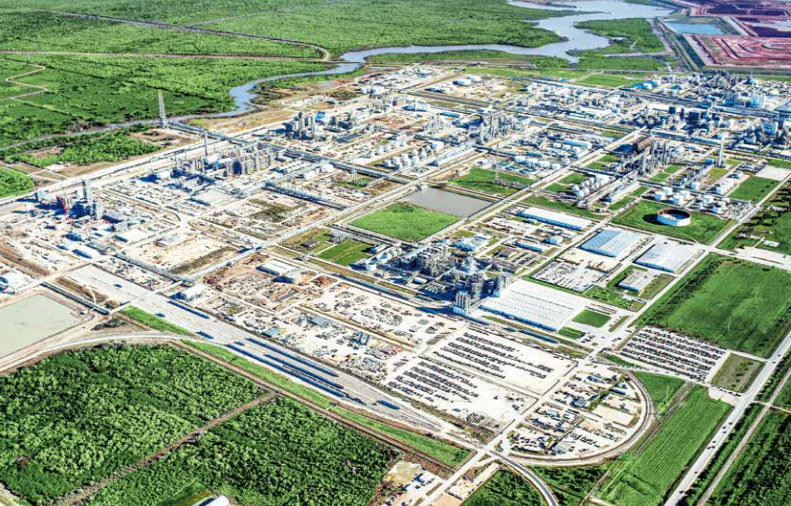
Aerial Bird View of Point Comfort Complex, TX
